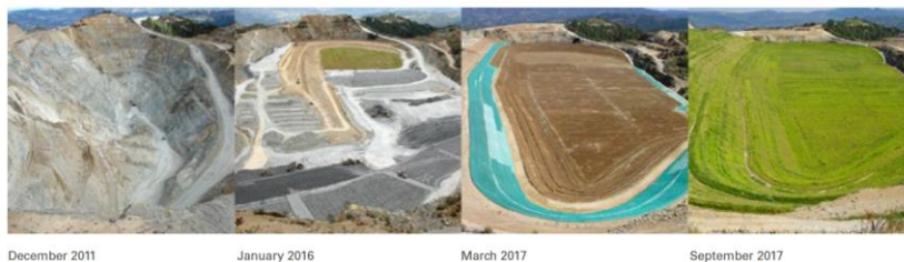
Figure 1 | Goldcorp's Marlin mine open pit closure
