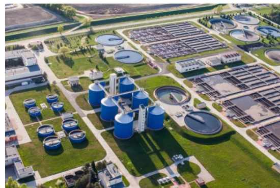
Figure 4 – Wastewater treatment plant
